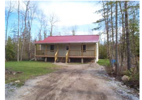
$159,900 Brand New Bungalow Desirable east side with access to calm waters on private beach
